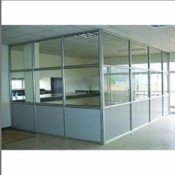
Aluminium Office Partition Fabrication Service
